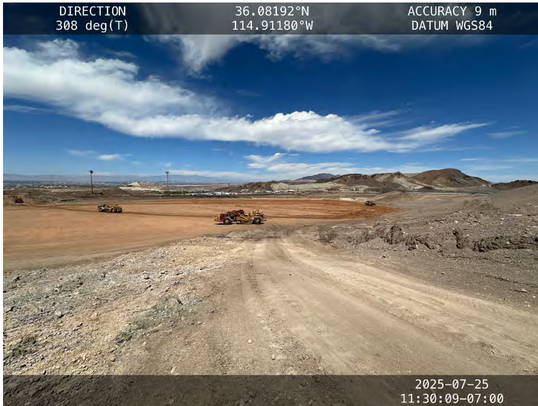
Hydro Pit silt layer placement – July 25, 2025
