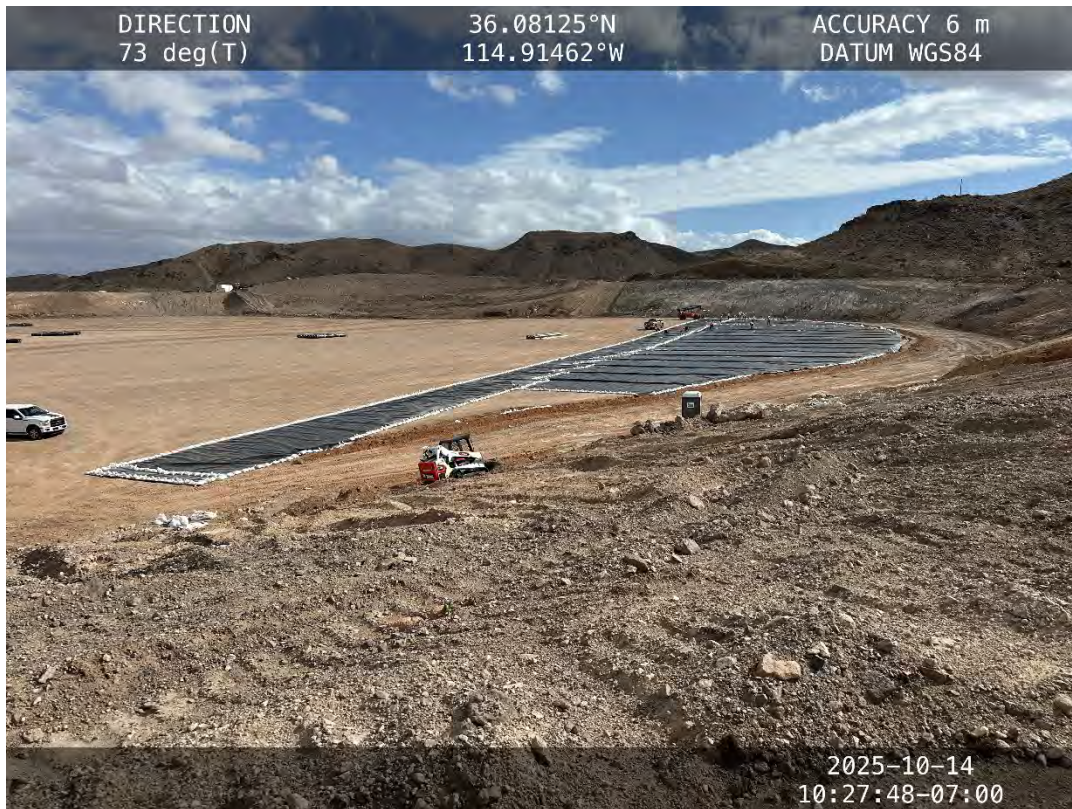
Hydro Pit liner installation – October 14, 2025
