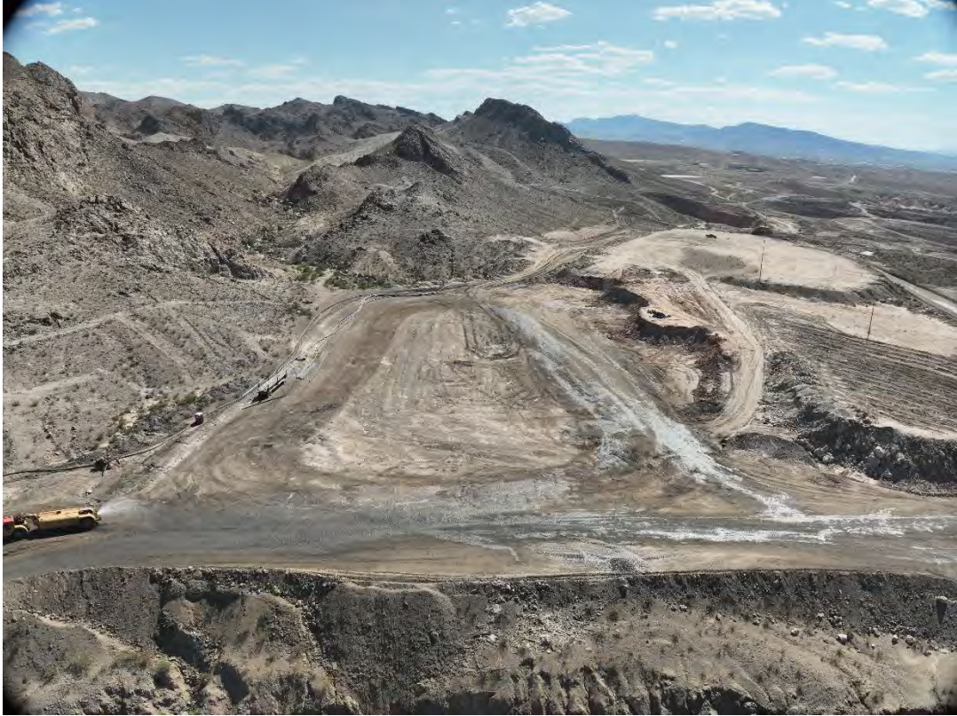
Tailings Stockpile area – September 4, 2025
