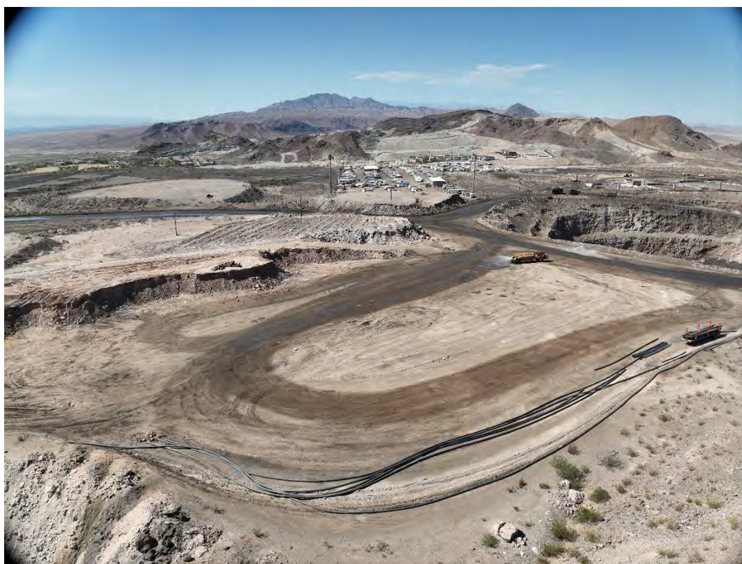
Tailings Stockpile area – September 4, 2025
