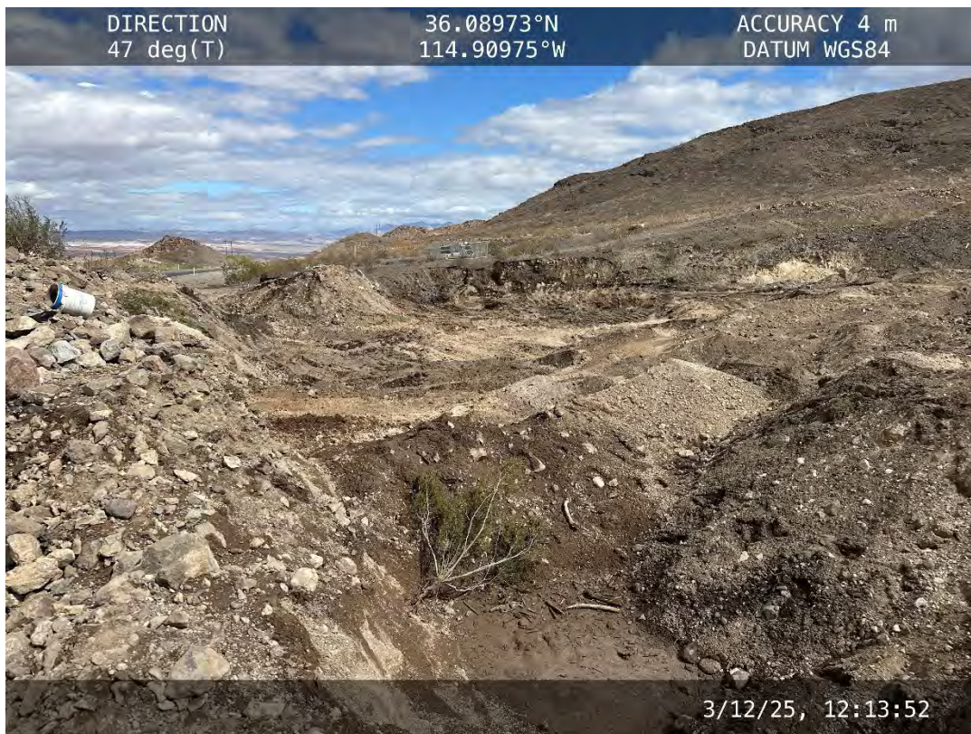
Northeast drainage – March 12, 2025
