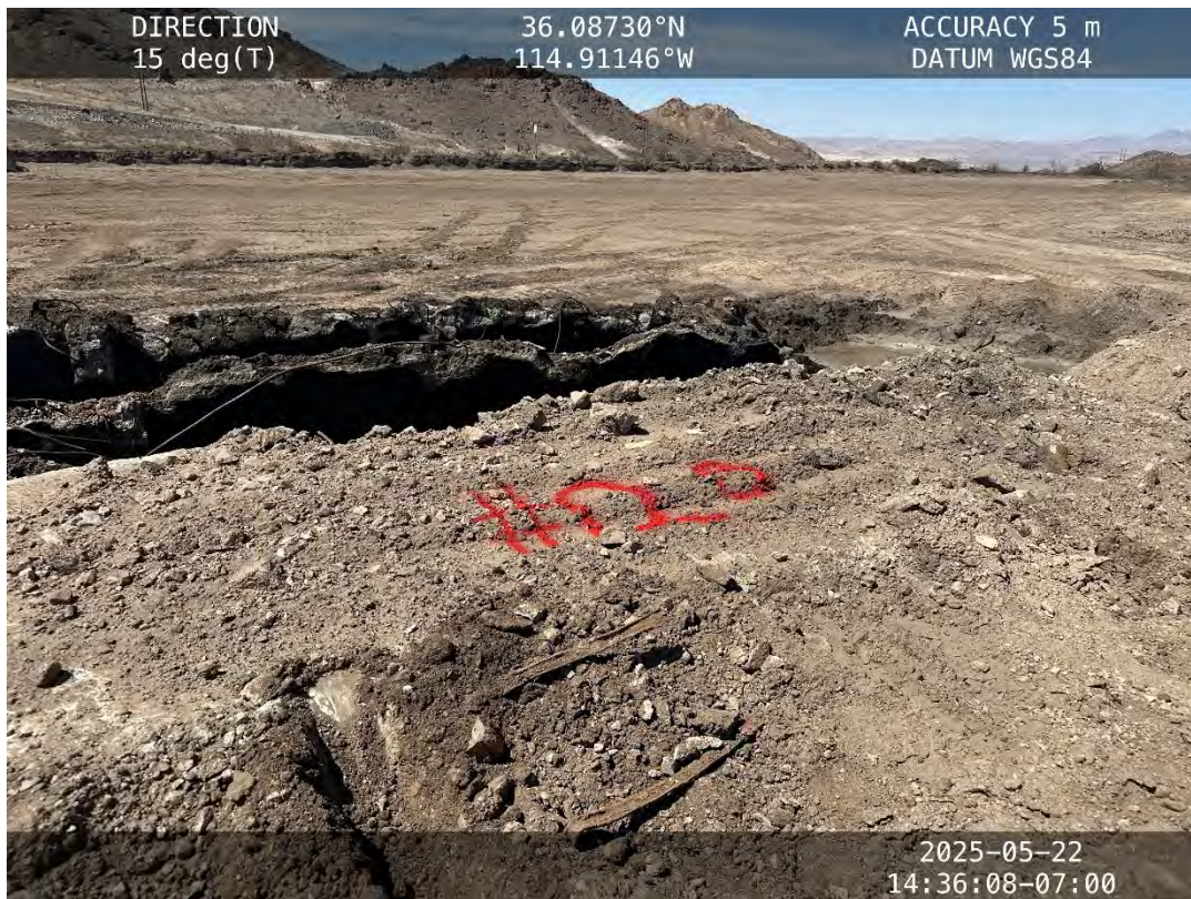
Location #12 – Concrete wall (east end)
