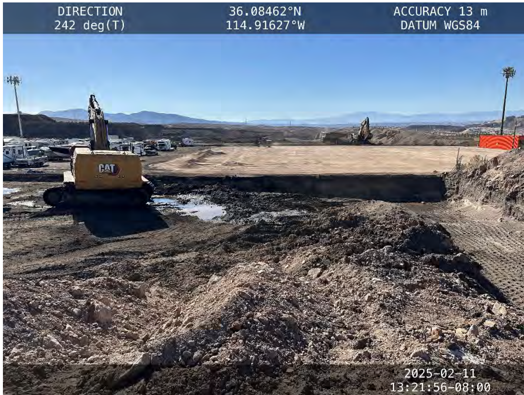
Tailings at Laker Plaza corner – February 11, 2025
