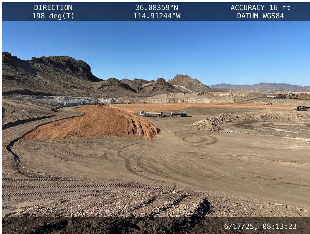
Hydro Pit silt layer placement – June 17, 2025
