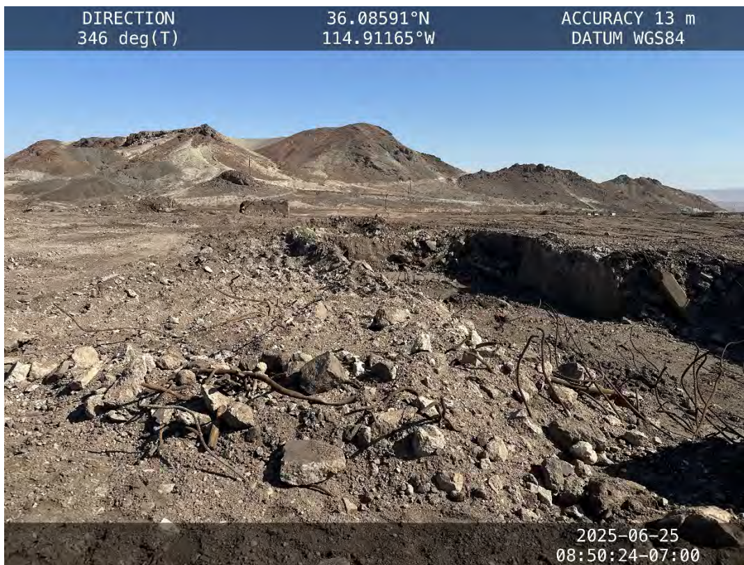
Location #34 - Concrete foundation
