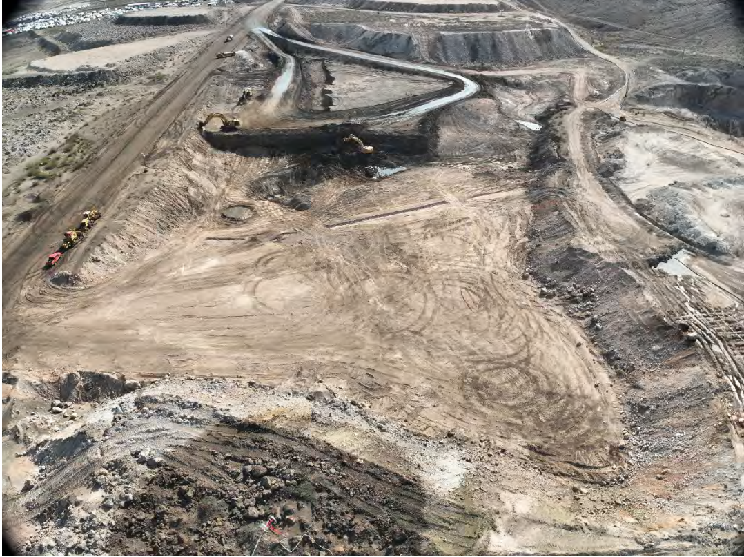
Tailings Pond 3 West – July 25, 2024
