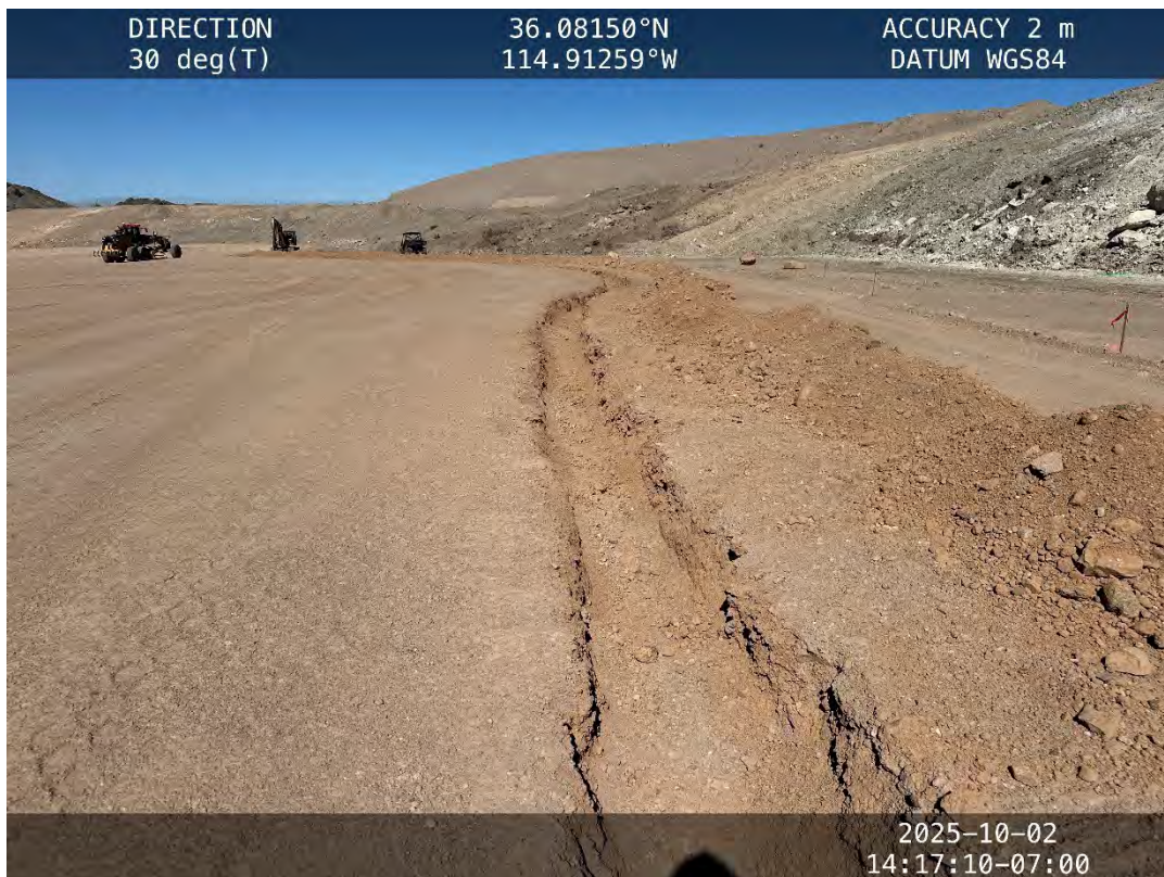
Hydro Pit anchor trench installation – October 2, 2025
