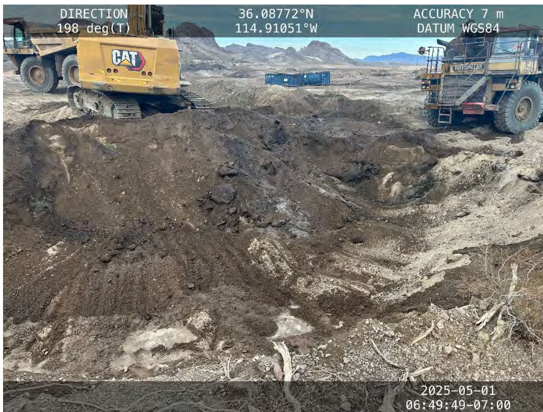
Fuel farm excavation – May 1, 2025
