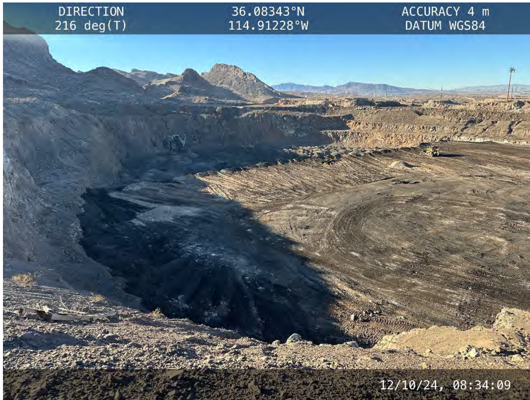
Hydro Pit Backfill – December 10, 2024
