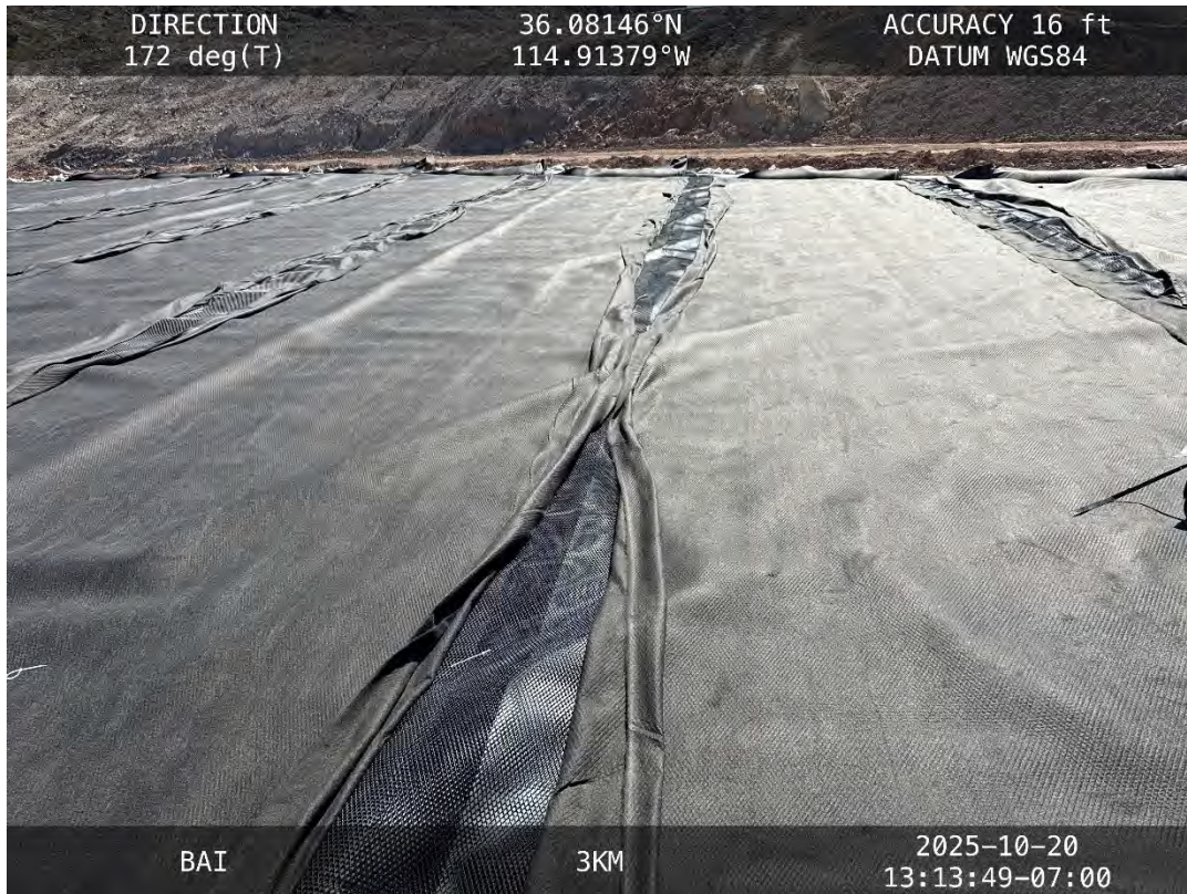
Drainage net and geotextile fabric installation over Hydro Pit liner – October 20, 2025
