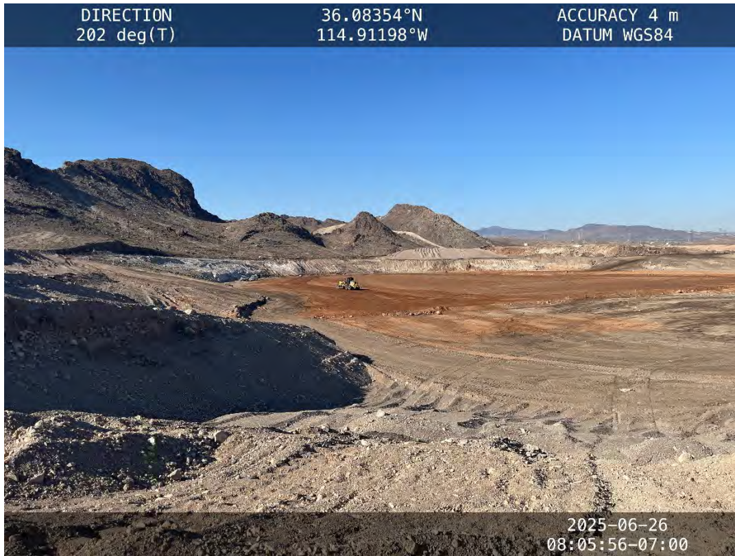
Hydro Pit silt layer placement – June 26, 2025
