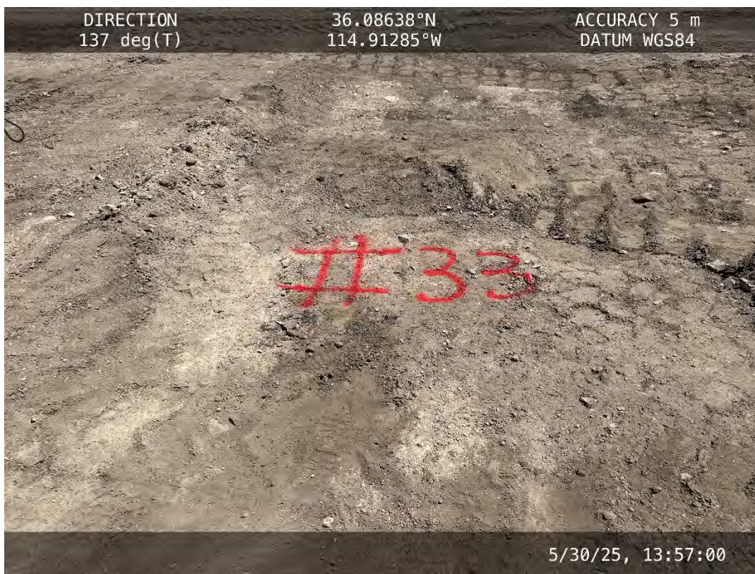
Location #33 – Concrete pad
