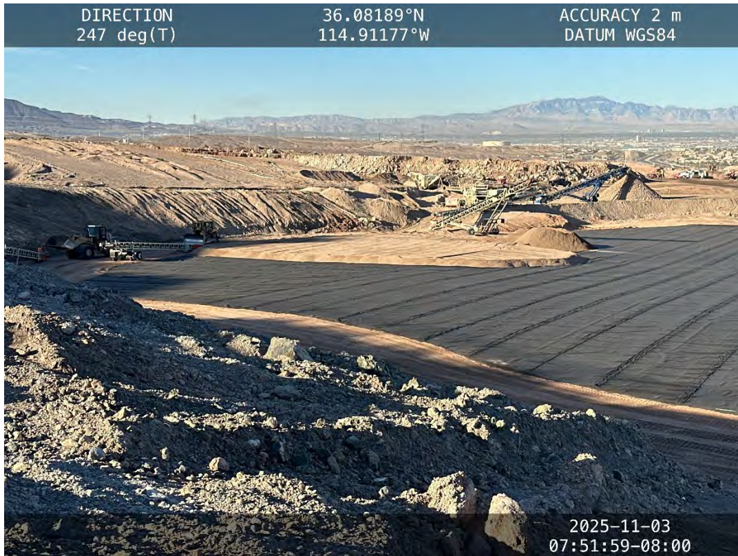
Cover placement over Hydro Pit liner – November 3, 2025
