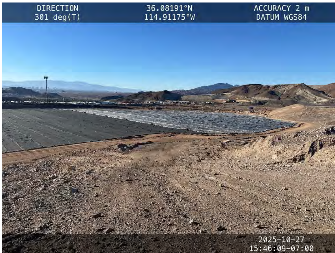
Hydro Pit liner installation – October 27, 2025
