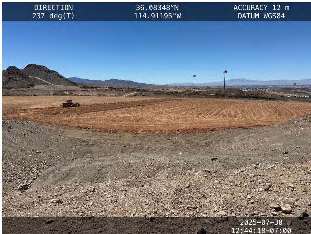
Hydro Pit silt layer placement – July 30, 2025
