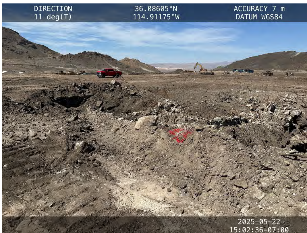
Location #15 – Concrete foundation
