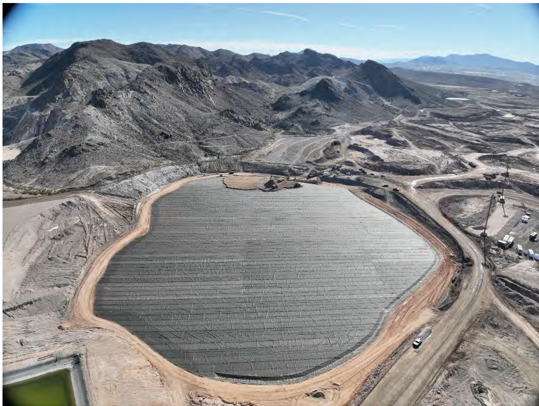
Completed Hydro Pit liner with cover placement – November 3, 2025
