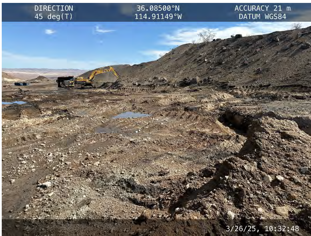
Tailings removal from Mill Site southeast of flotation cells – March 26, 2025
