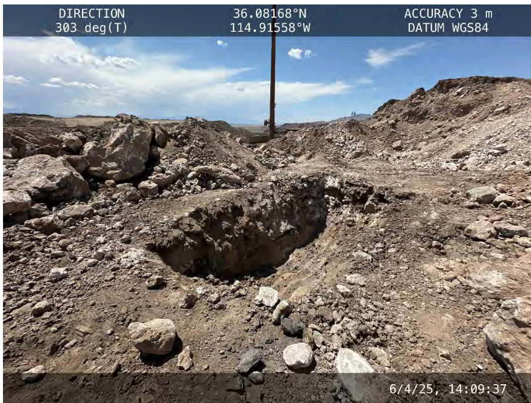
Tailings seam southeast of Tailings Pond 1 – June 4, 2025
