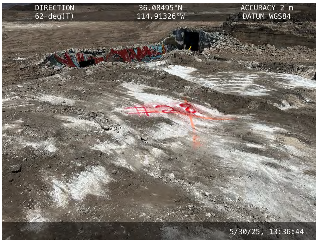
Location #28 – Concrete pad
