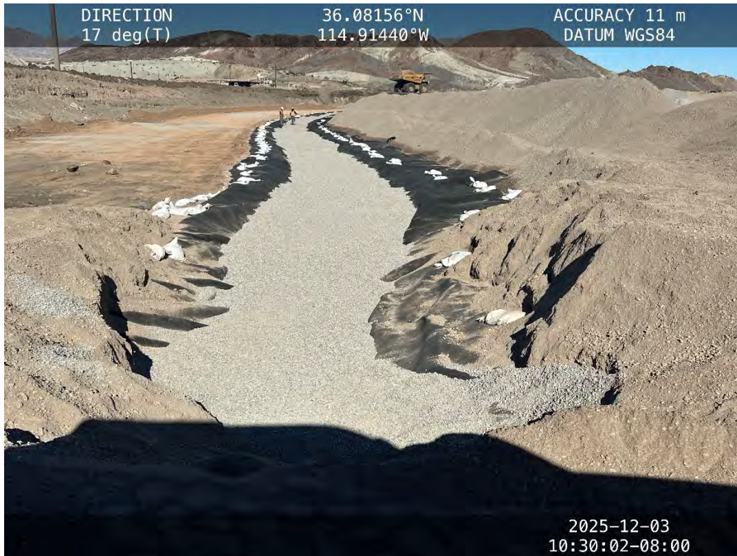
Hydro Pit drainage channels backfilled with Zone 3 material – December 3, 2025
