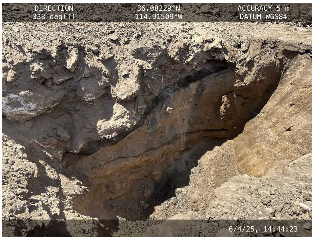
Tailings seam southeast of Tailings Pond 1 – June 4, 2025
