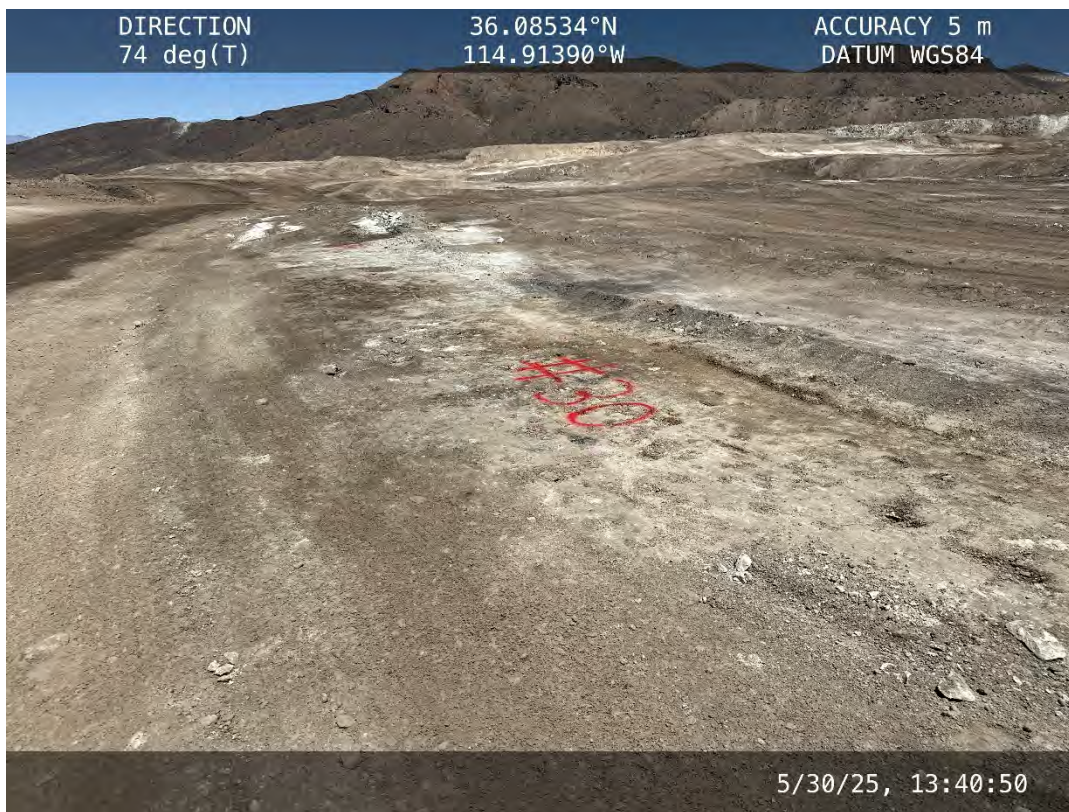
Location #30 – Concrete pad
