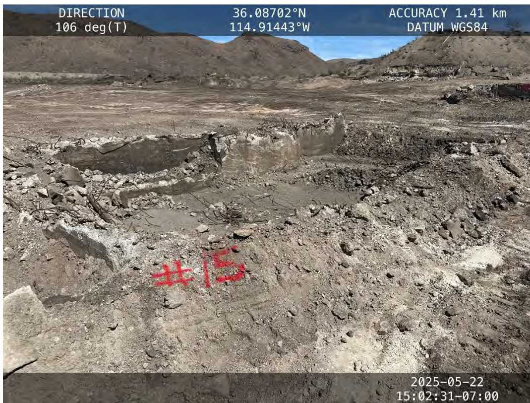
Location #15 – Concrete foundation
