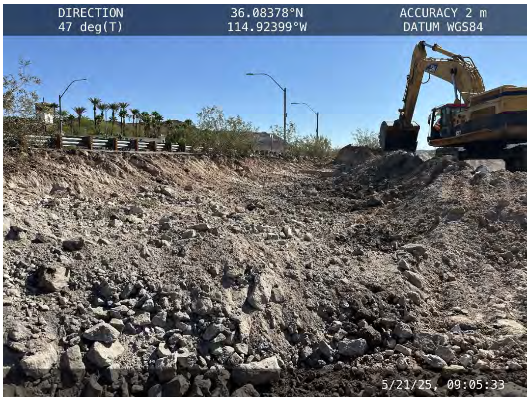
Tailings from north end of Closure Unit 3b/Development Area 4 – May 21, 2025
