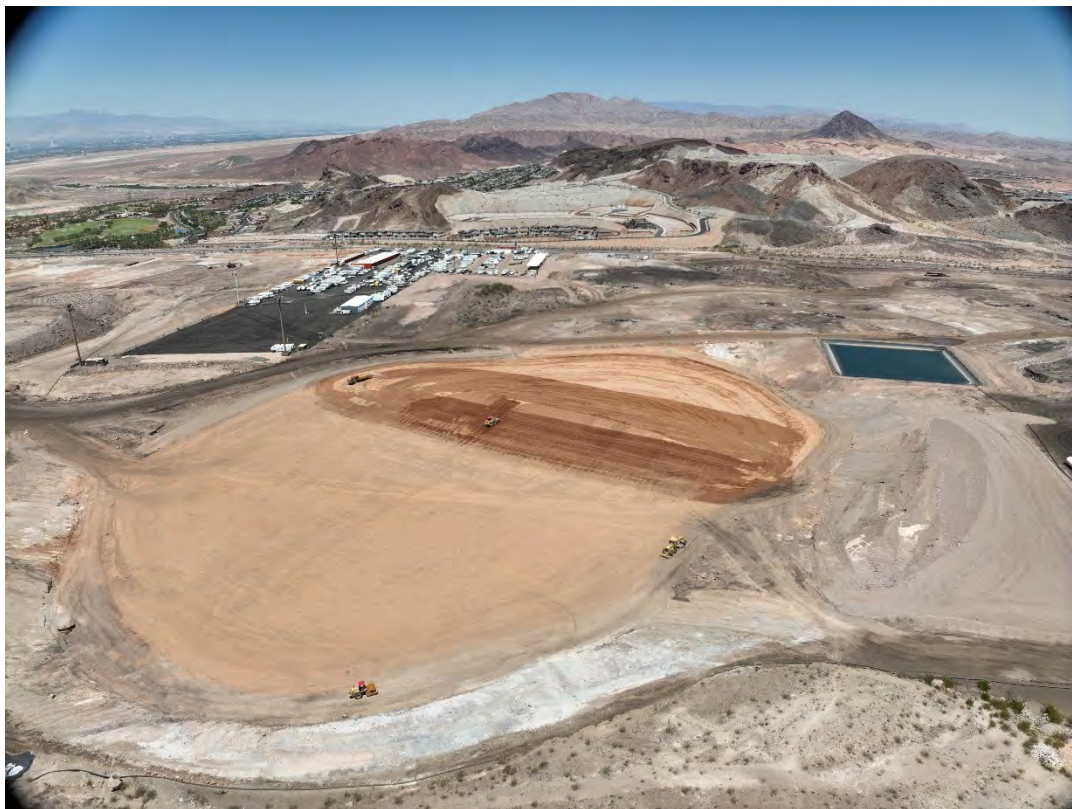
Hydro Pit backfill with silt layer – July 24, 2025
