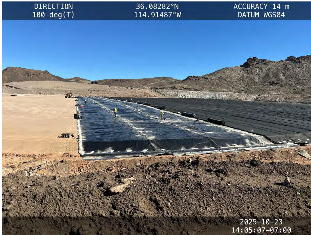
Hydro Pit liner installation – October 23, 2025
