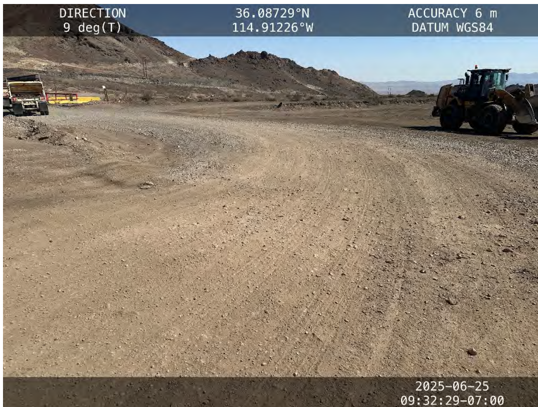
Location #37 – Haul road constructed over excavation area with track-out rock
