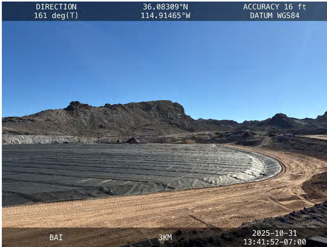
Completed Hydro Pit liner with cover placement – October 31, 2025
