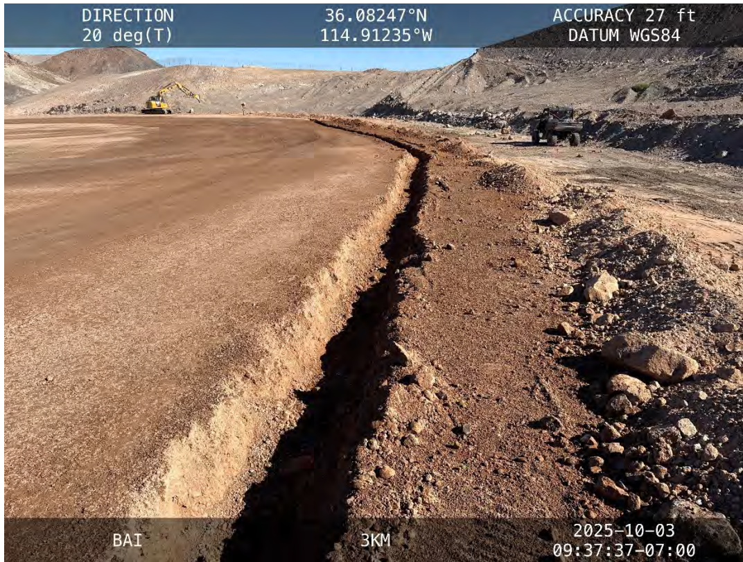
Hydro Pit anchor trench installation – October 3, 2025
