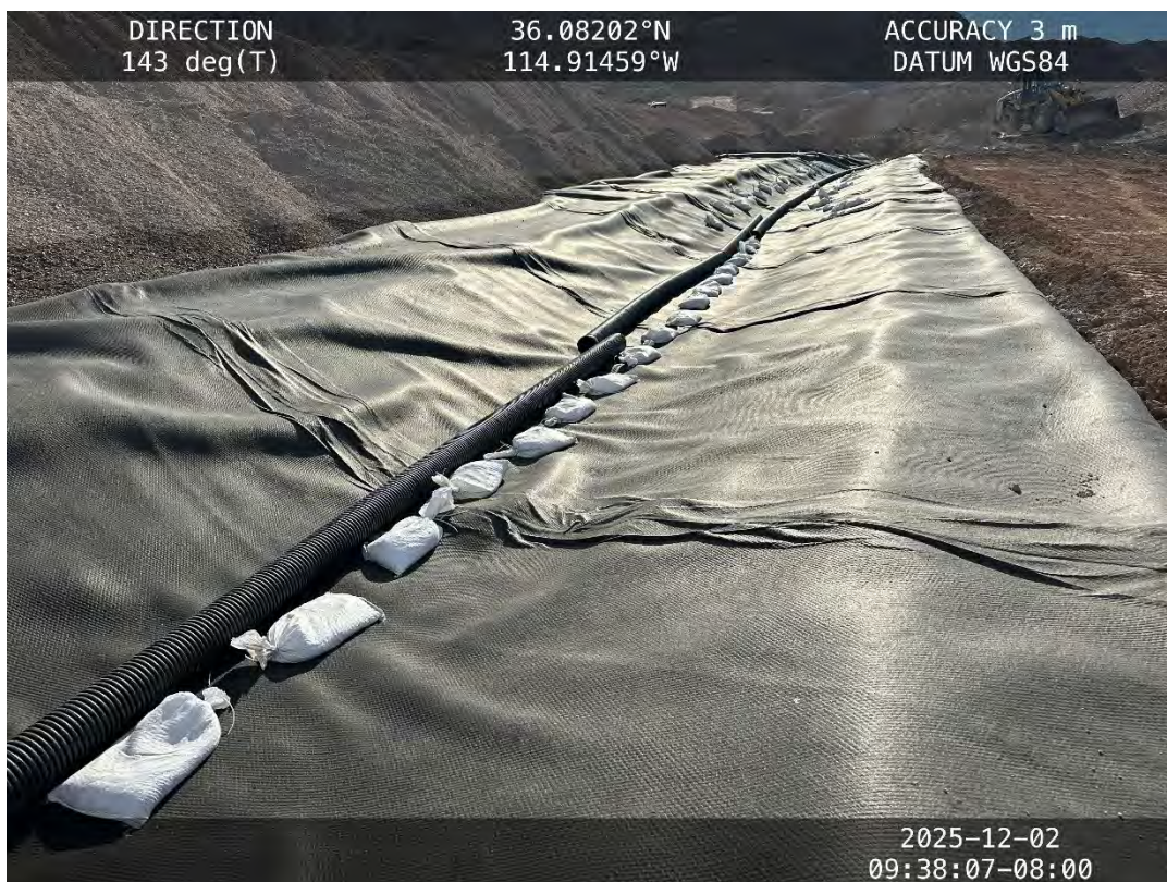
Hydro Pit drainage channel perforated pipe installation – December 2, 2025
