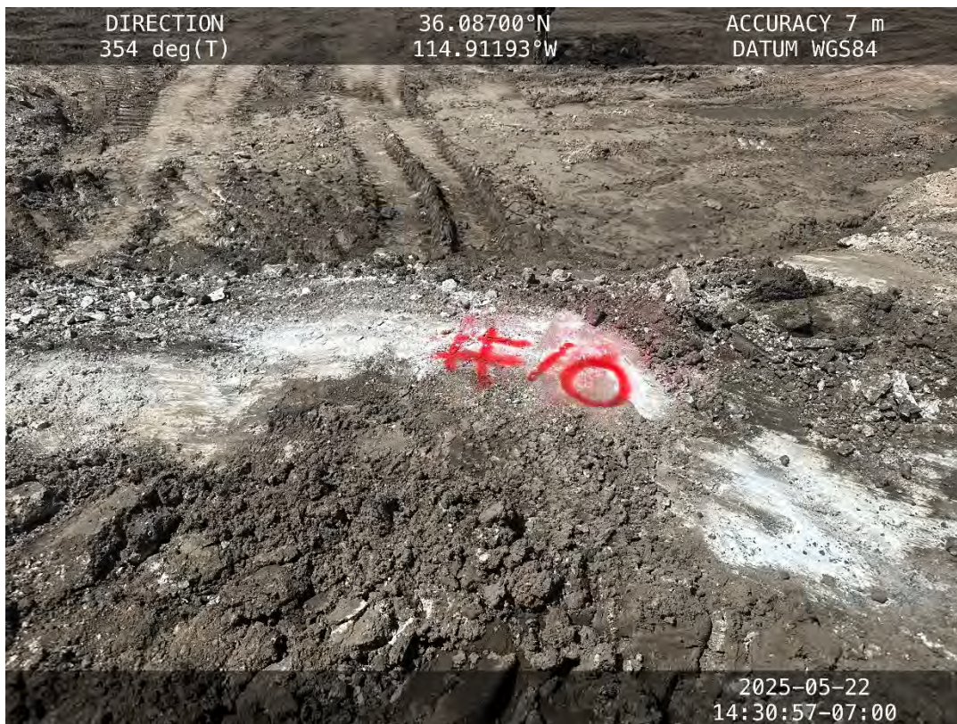
Location #10 – Hard material, concrete or gypsum bedrock
