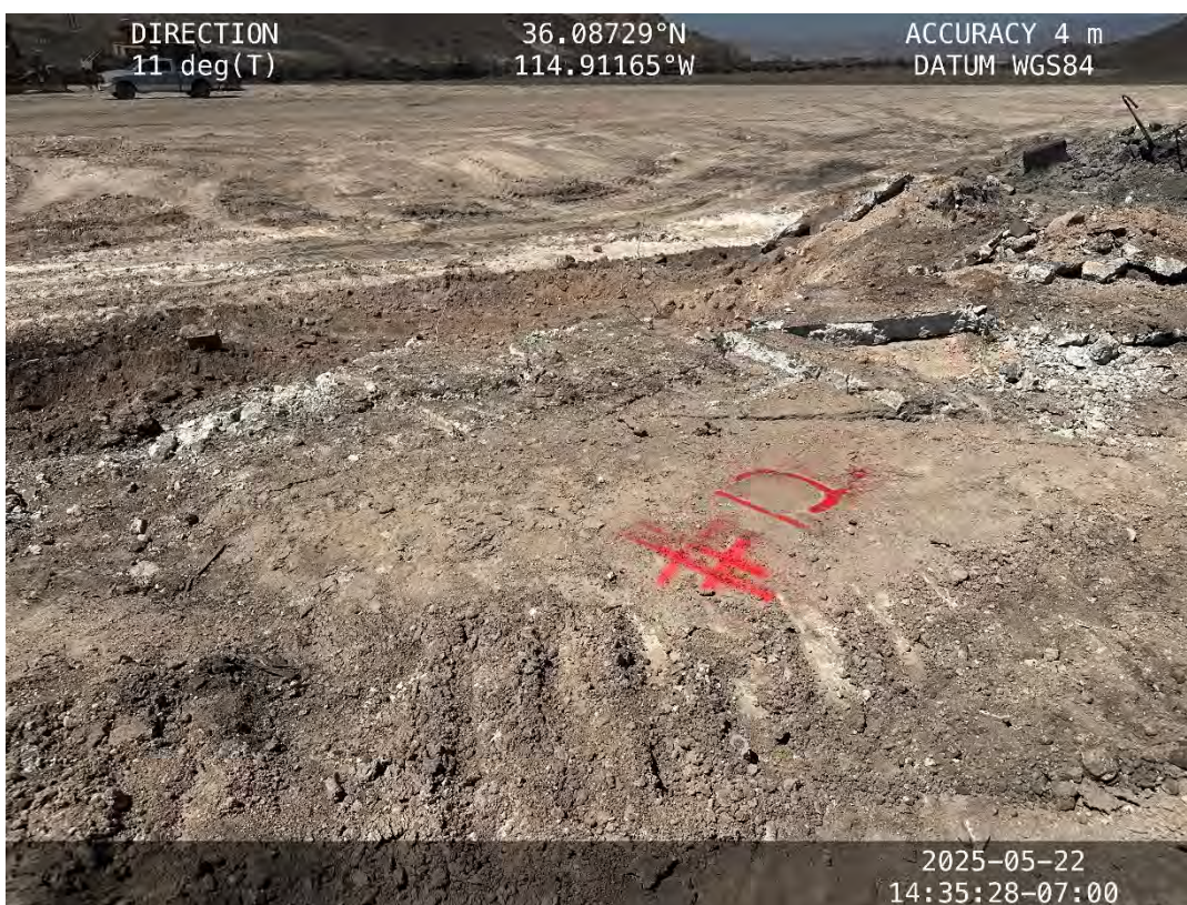
Location #12 – Concrete wall (west end)
