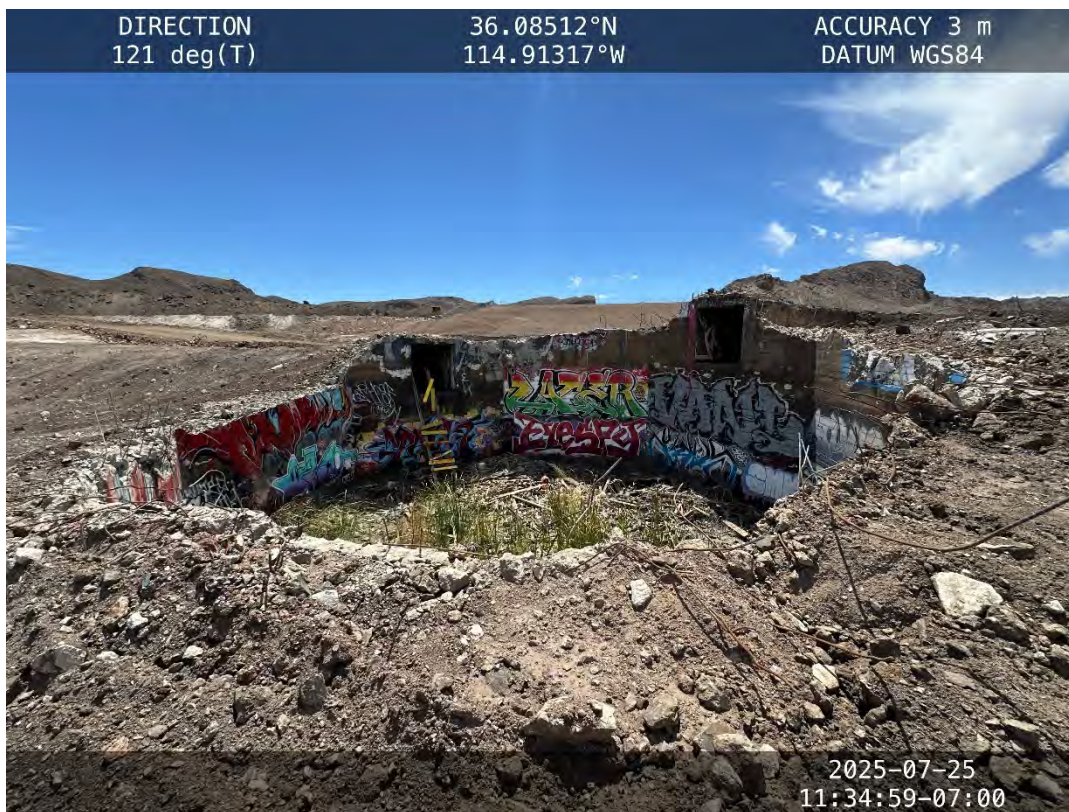
Location #22 – Western octagonal sump structure
