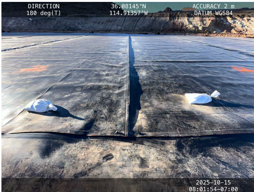
Hydro Pit liner installation – October 15, 2025
