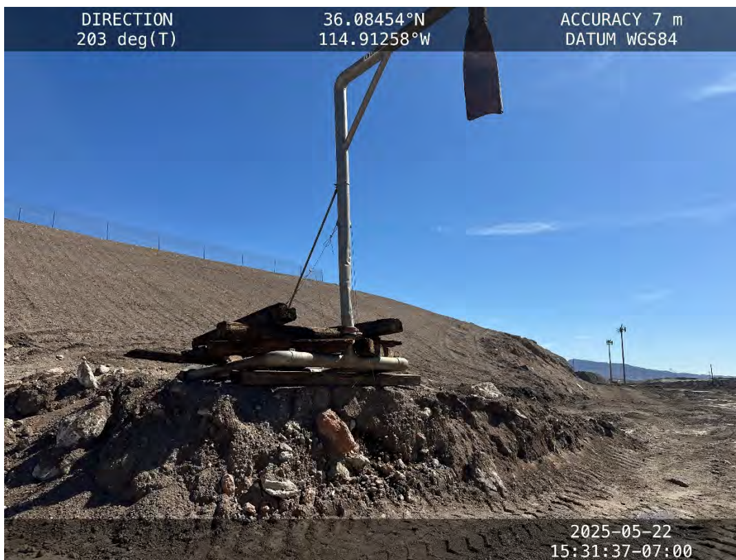
Location #19 – Slope containing construction water pond and J-stand
