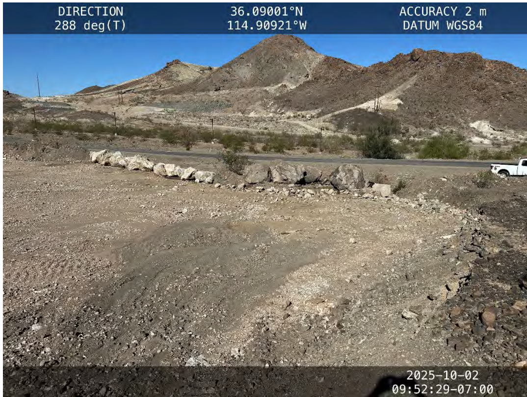
Northeast drainage – October 2, 2025
