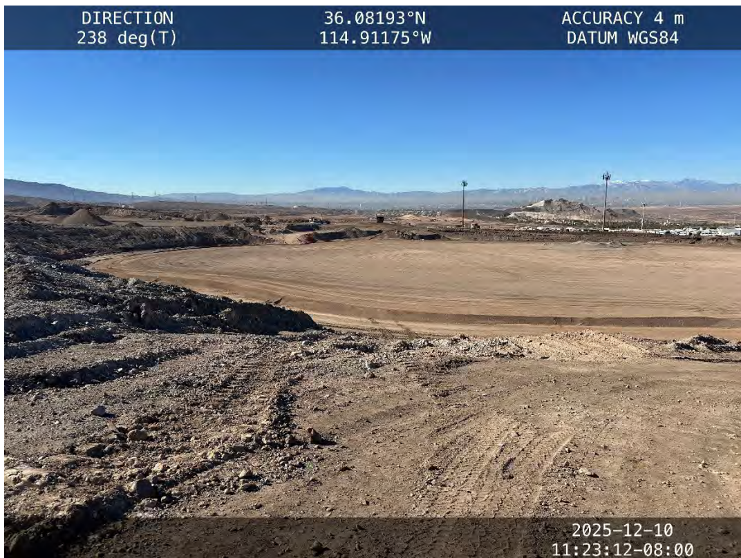
Two-foot cover over Hydro Pit liner – December 10, 2025
