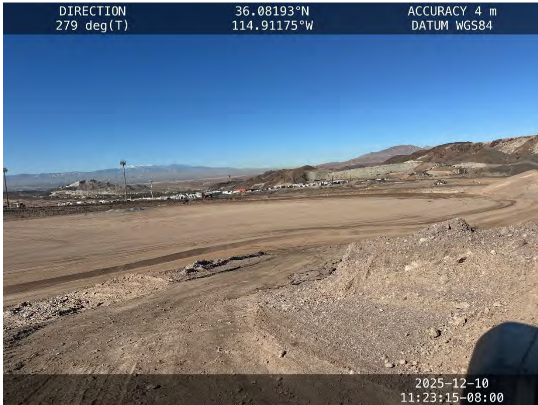
Two-foot cover over Hydro Pit liner – December 10, 2025
