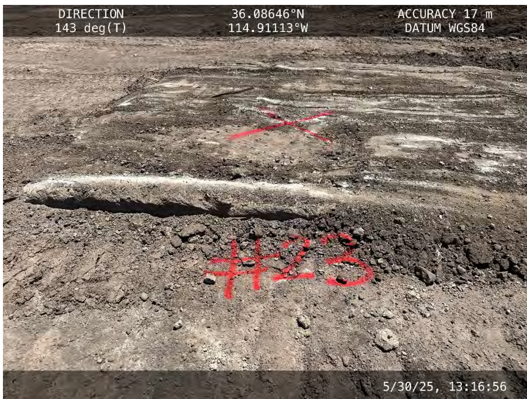
Location #23 – Concrete pad
