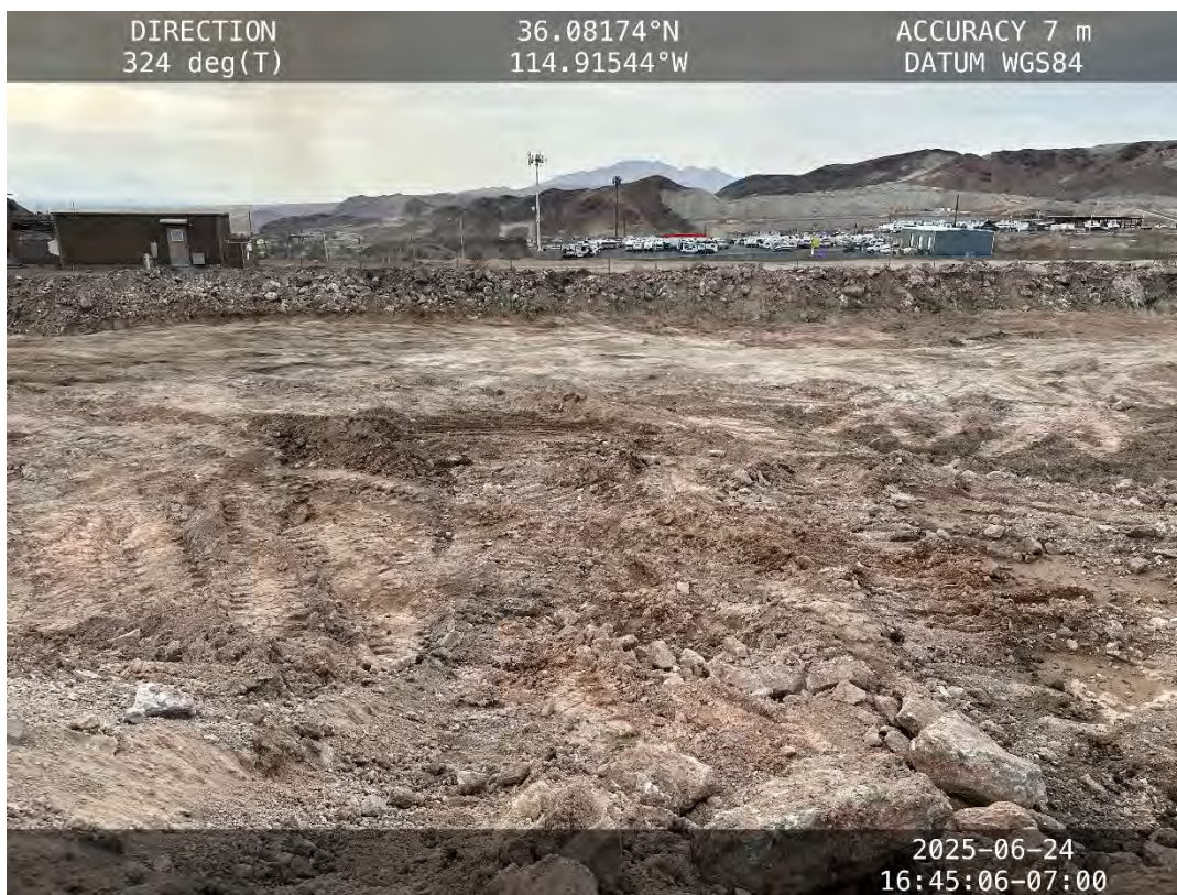
Cleared area from tailings seam southeast of Tailings Pond 1 – June 24, 2025
