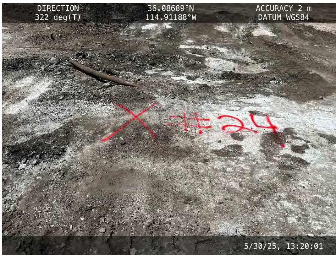
Location #24 – Concrete pad
