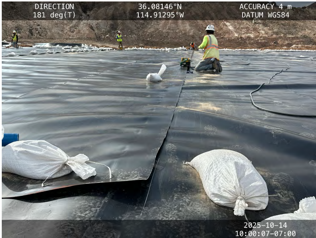
Hydro Pit liner installation – October 14, 2025
