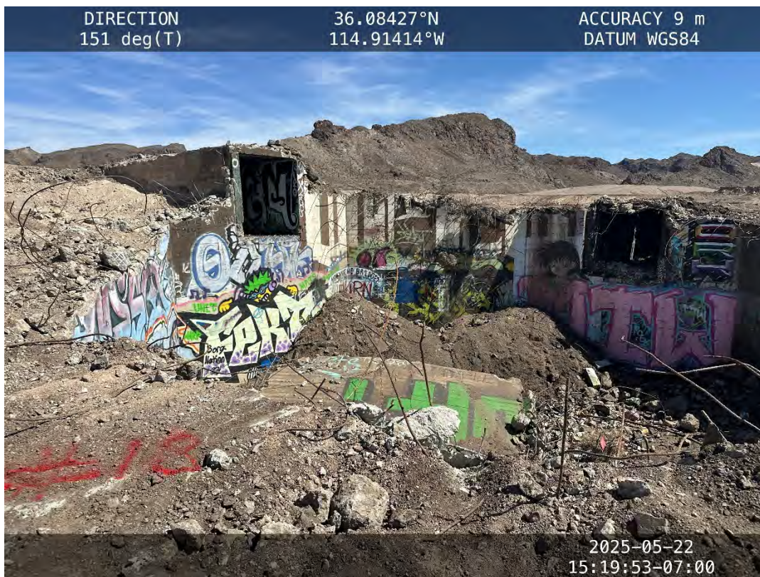
Location #18 – Western octagonal sump structure
