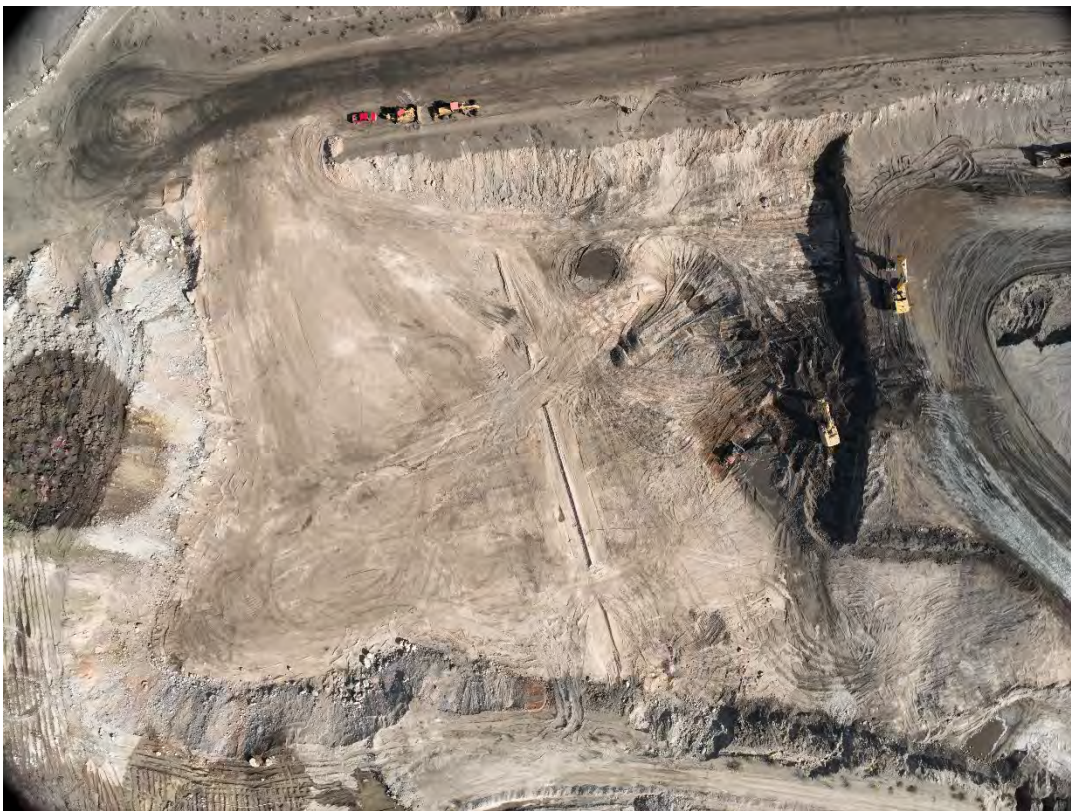
Tailings Pond 3 West – July 25, 2024
