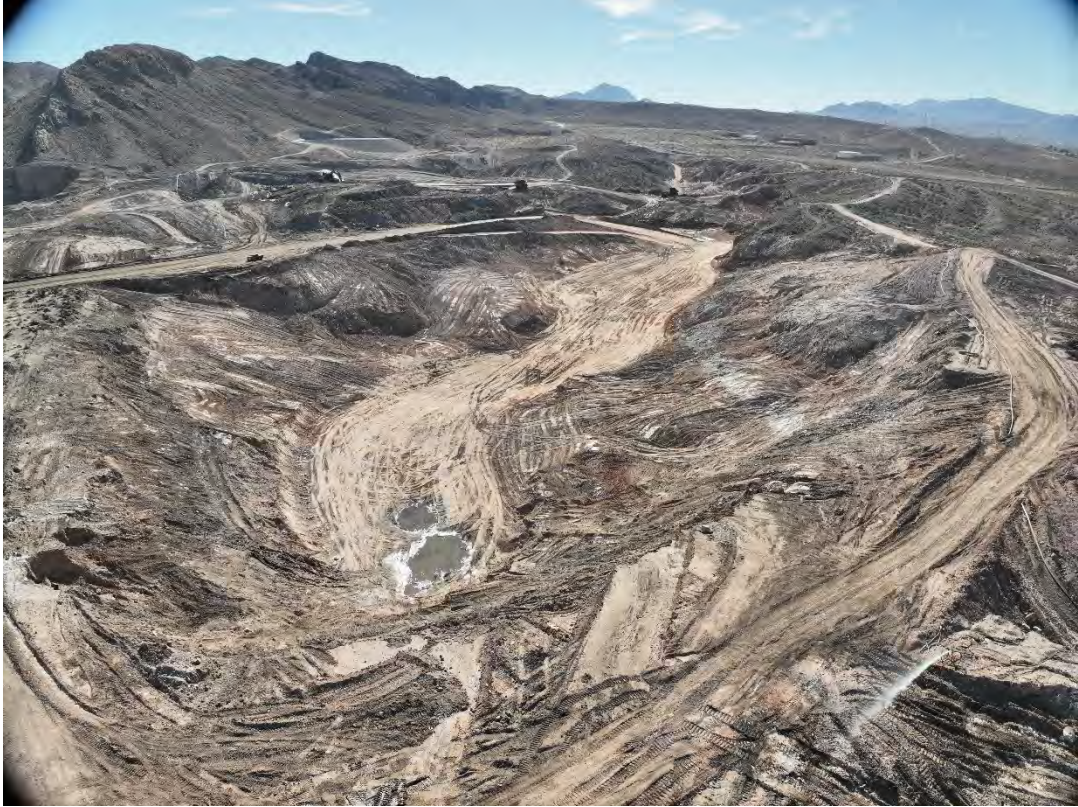
Tailings Pond 2 North – November 18, 2024
