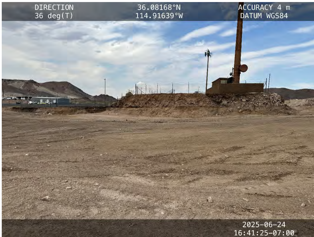
Cleared area from tailings seam southeast of Tailings Pond 1 – June 24, 2025
