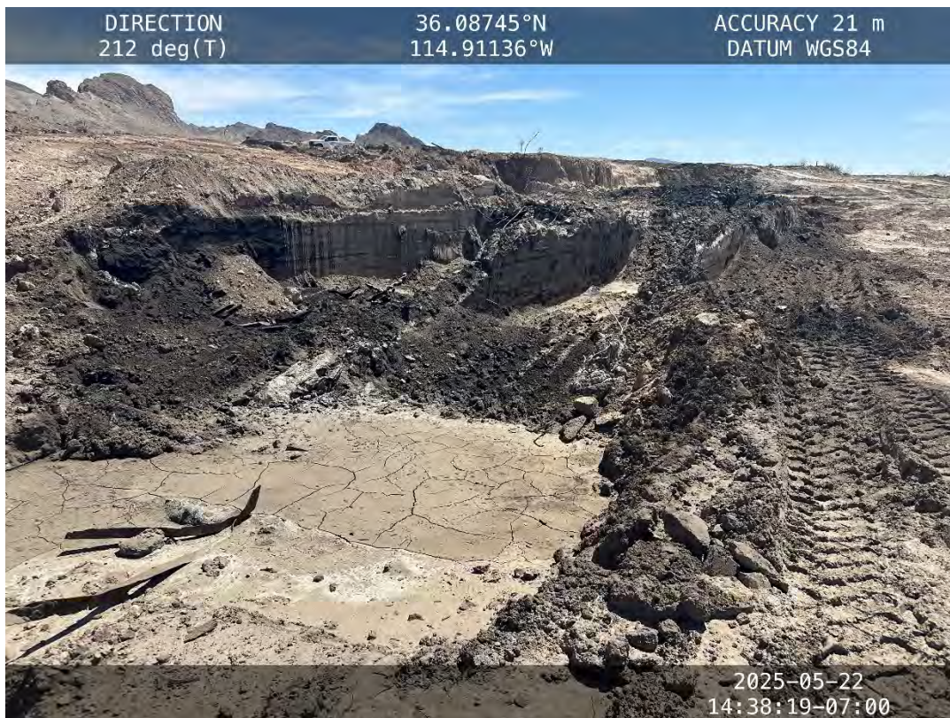
Location #12 – Concrete wall
