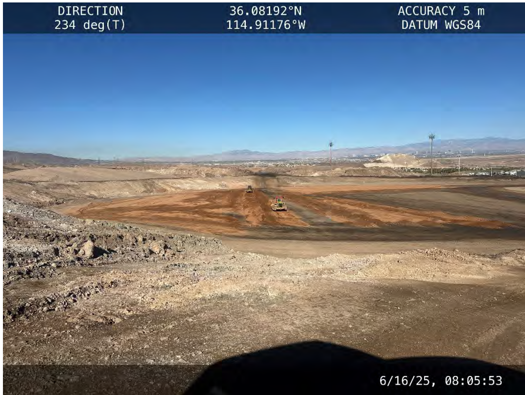
Hydro Pit silt layer placement – June 16, 2025
