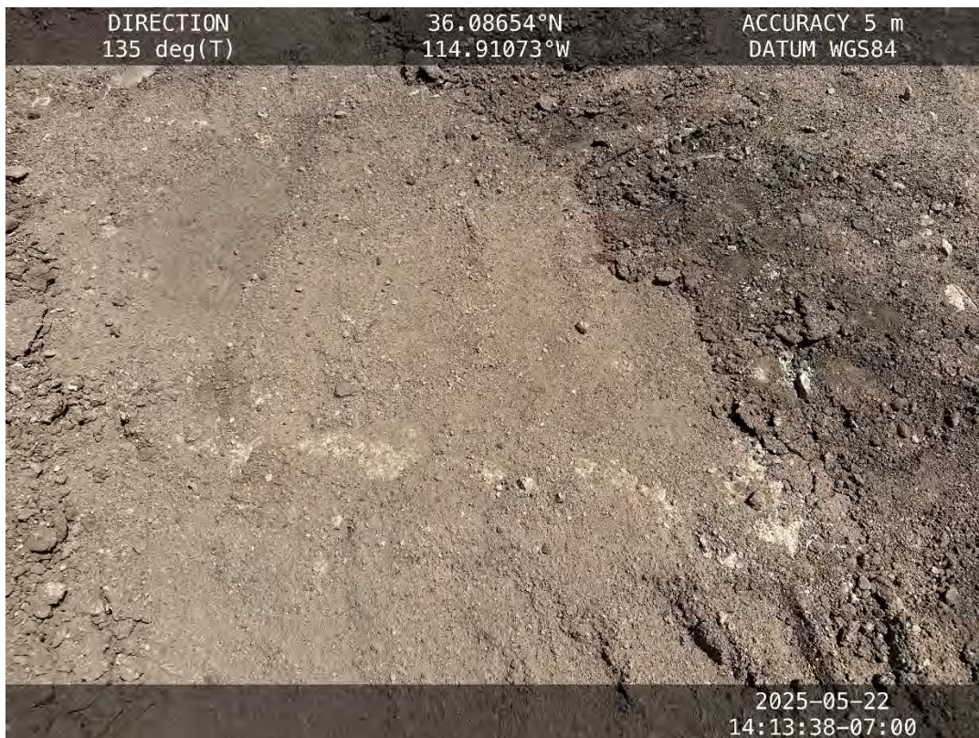
Location #2 – Concrete pad
