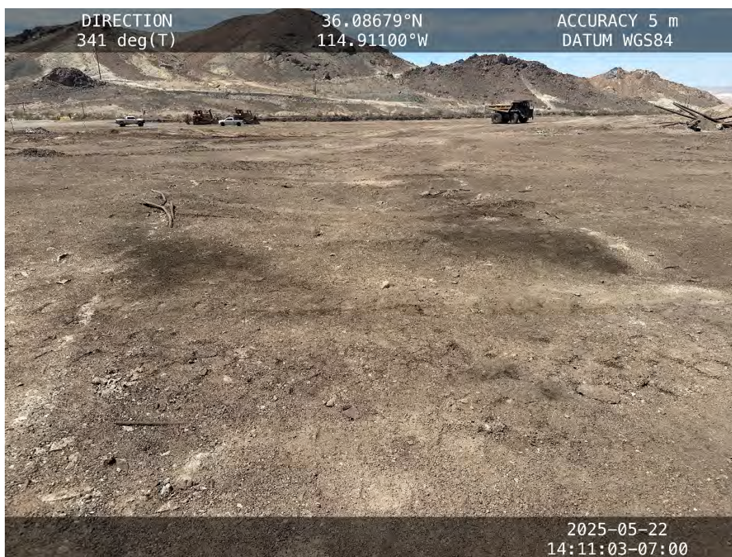
Location #1 – Concrete pad
