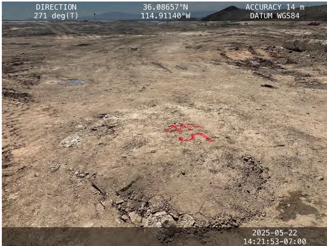
Location # 5 – Concrete pad
