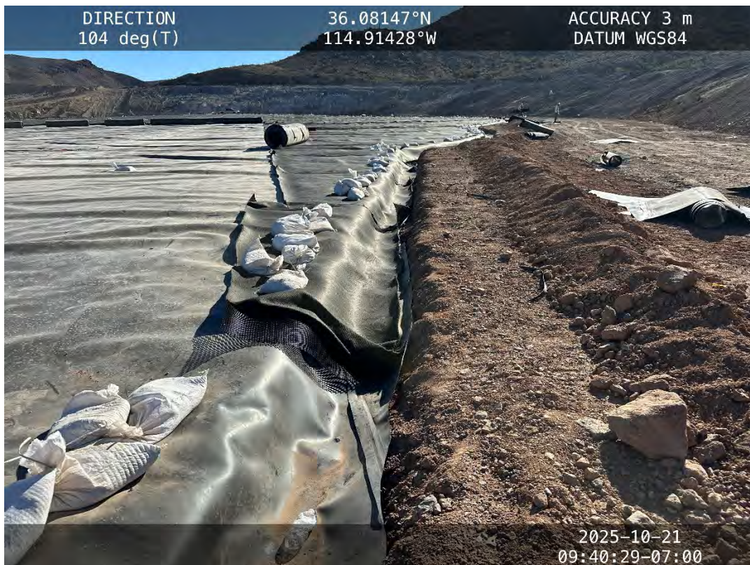
Drainage net and geotextile fabric installation over liner at anchor trench – October 21, 2025
