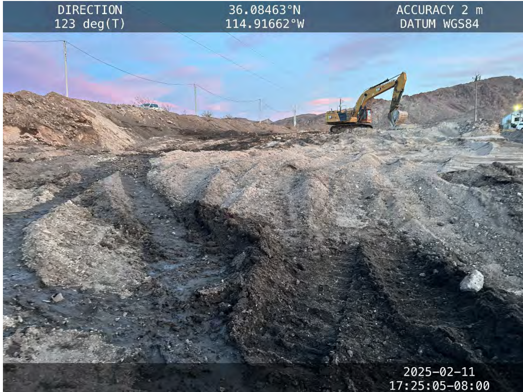
Laker Plaza corner after tailings removal – February 11, 2025
