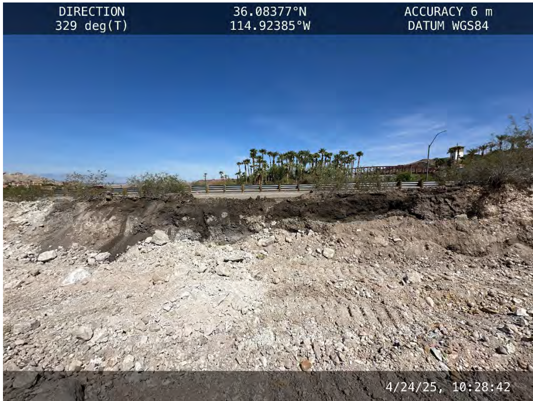
Tailings from north end of Closure Unit 3b/Development Area 4 – April 24, 2025
