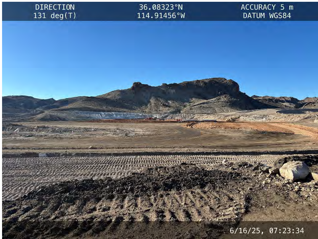
Hydro Pit silt layer placement – June 16, 2025
