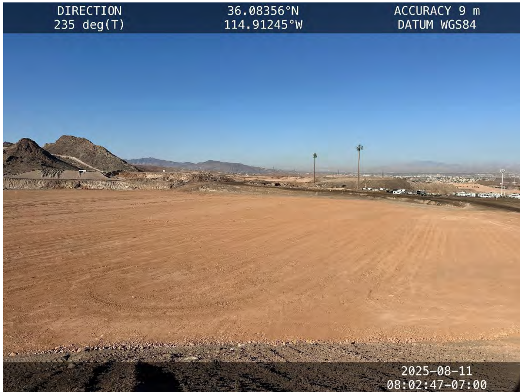
Hydro Pit silt layer completed – August 11, 2025
