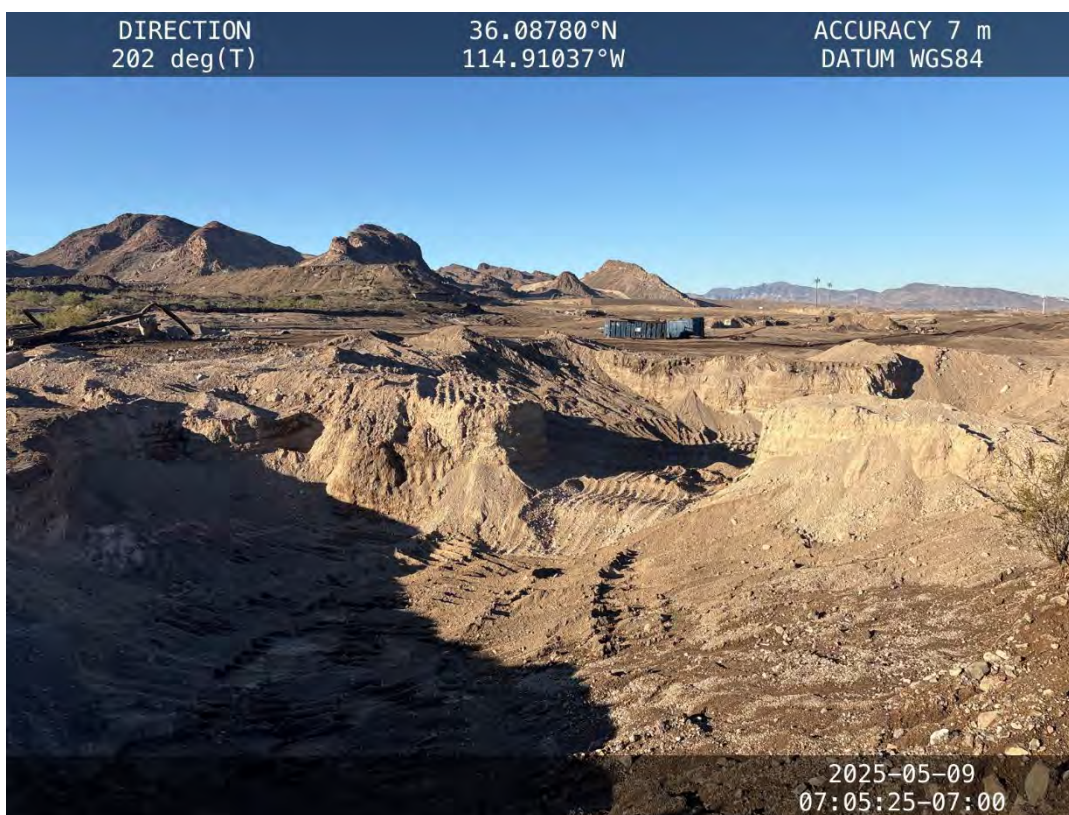
Fuel farm excavation – May 9, 2025
